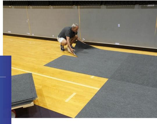
100% Recycled Polyester Topcloth Tri-Layer Extruded Backing with Moisture Barrier Floor Surface
